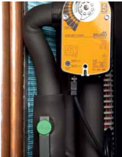
2-way/3-way valve changeover
