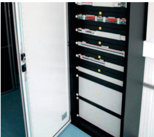
Power distribution cabinet with automatic transfer switch (ATS) from Asco, another division of Emerson Network Power.
